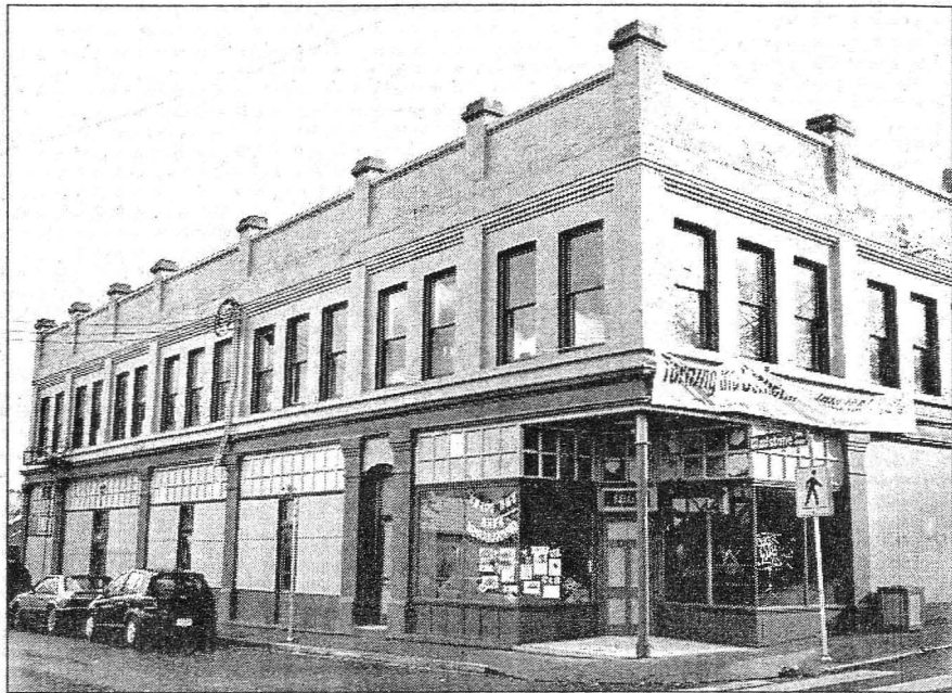
The Fernwood Community Centre Society is getting a $50,000 city grant to help build affordable suites in this empty building. Bruce Stotesbury/Times Colonist
