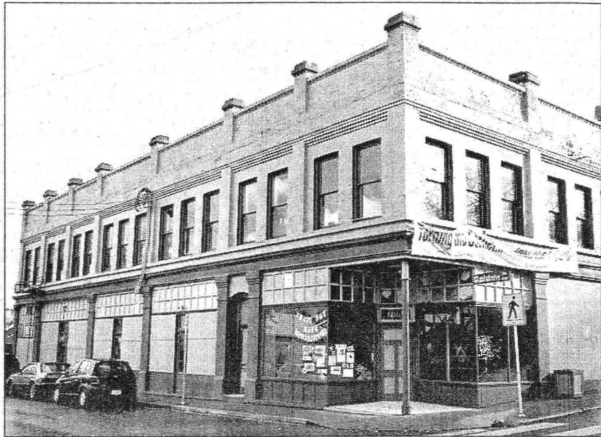
The Fernwood Community Centre Society is getting a $50,000 city grant to help build affordable suites in this empty building. Bruce Stotesbury/Times Colonist
